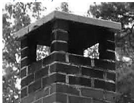
Concrete Cap Chimney Top
